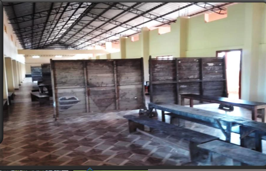
St.Mary’s Boys High School, Alappuzha, Kerala: Construction of School Building
